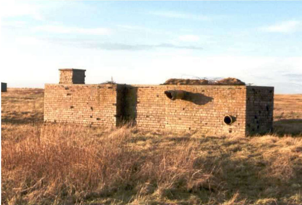
Figure 15 RAF Castletown's Q site control building
