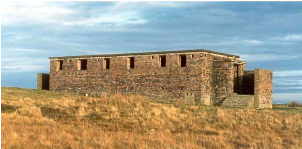
Figure 19 Combined transmitter / receiver building at Ulbster CHL radar station
