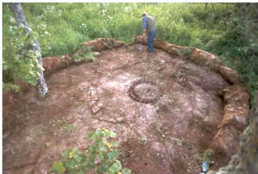
Figure 9 Concrete apron (left) with ring of mounting bolts in the centre, for the 4.7" gun installed at Castletown. The letters RAF (right) are set at the foot of the tree to the left.
