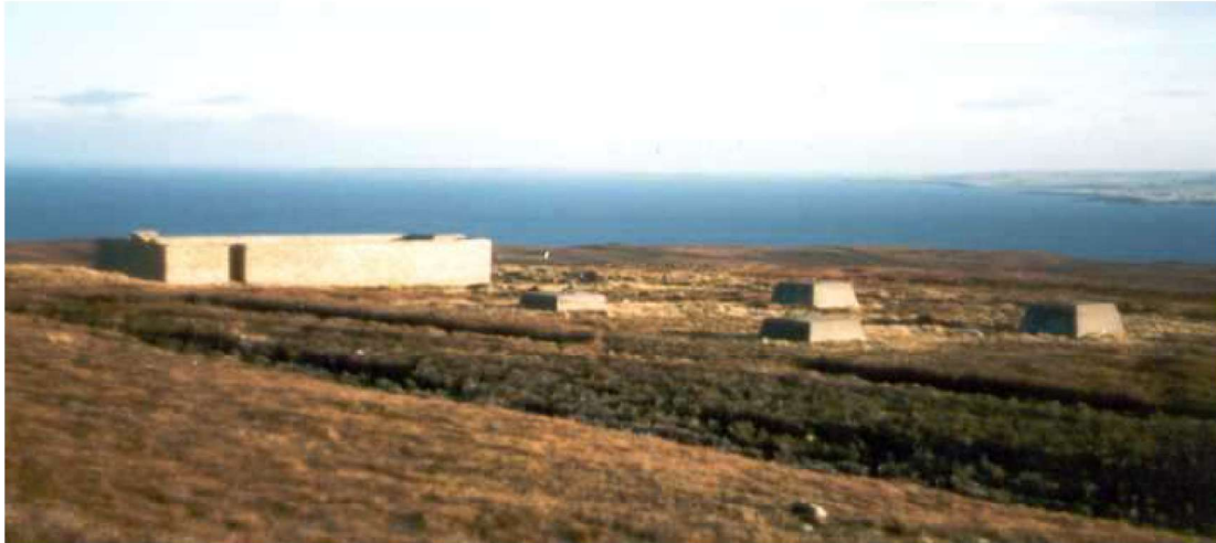
Figure 21 Blast walls protecting one of the transmitter huts at Burifa Hill. The four concrete footings for the 240 ft. wooden transmitter mast can be seen to the right.
