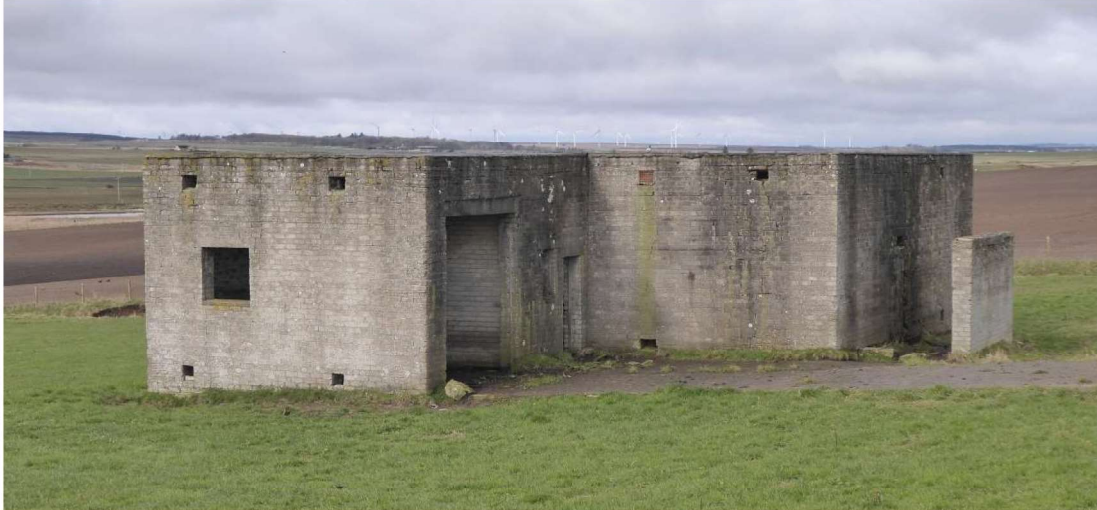
Figure 27 DTN building, with garage annex at left and blast wall protected entrance to right
