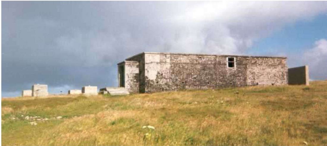
Figure 20 The identical building at Dunnet Head CHL radar station
