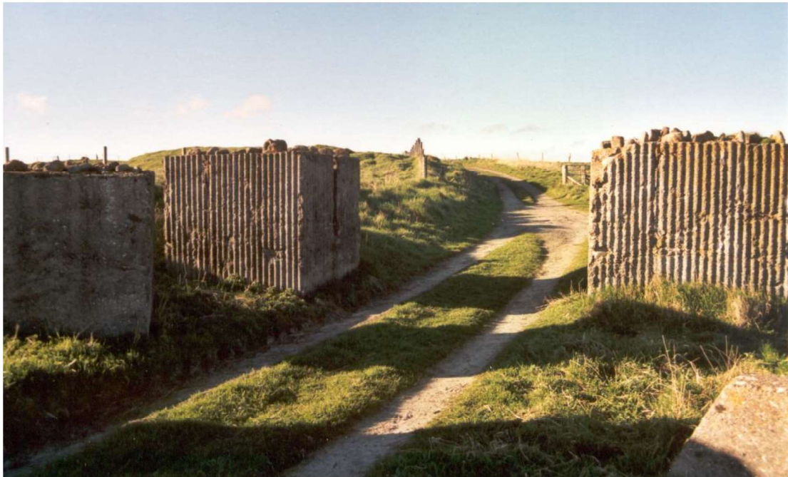
Figure 2 Road barrier at Freswick bay.
