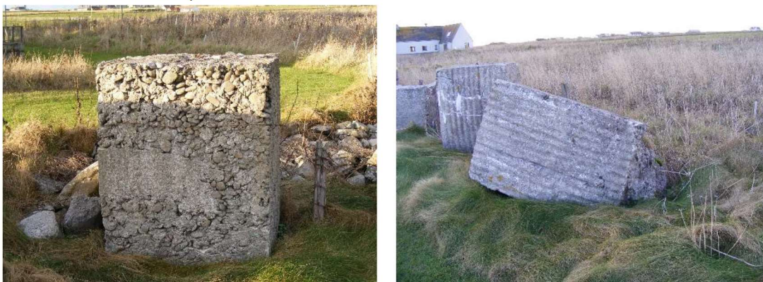
Figure 4 This anti-tank cube (left) shows the use of beach pebbles to eke out the cement. The foundation of the cube (right) is almost non-existent, this could have been easily pushed aside.
