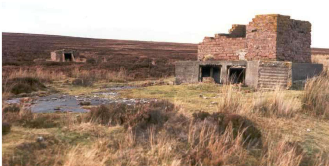
Figure 16 LAA emplacement at Tannach CH radar station.
