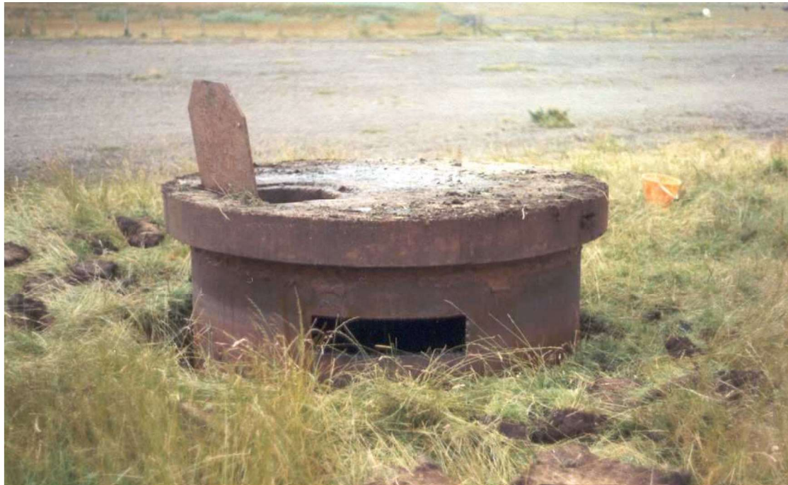
Figure 10 Pickett-Hamilton retractable fort at RAF Castletown, in raised position.
