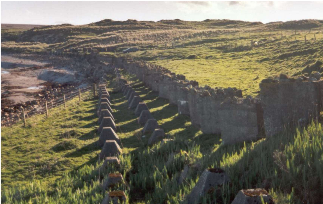
Figure 1 Anti-tank obstacles on Freswick Bay
