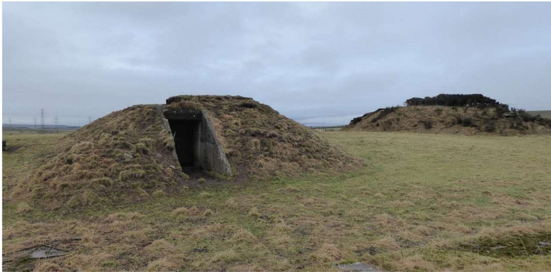
Figure 25 Hoy AFDD, with gas decontamination in foreground and pump room in distance
